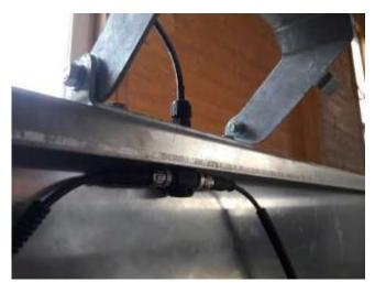
Connect the two weighing signal cables on the right and left to the distributor.
