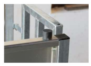
Attach the rubber buffer on the left-hand side panel, as shown.
